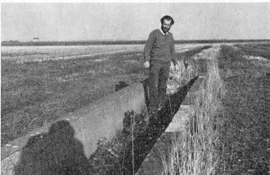
Top: Irrigation gun spraying digested sludge over one-third of an acre. Centre: Sewage is run into lagoons at 300,000 galls. per acre. When dry it is ploughed and cropped for five years. Bottom: Original 19th Century irrigation channels have been replaced, but the system still grows good crops.
