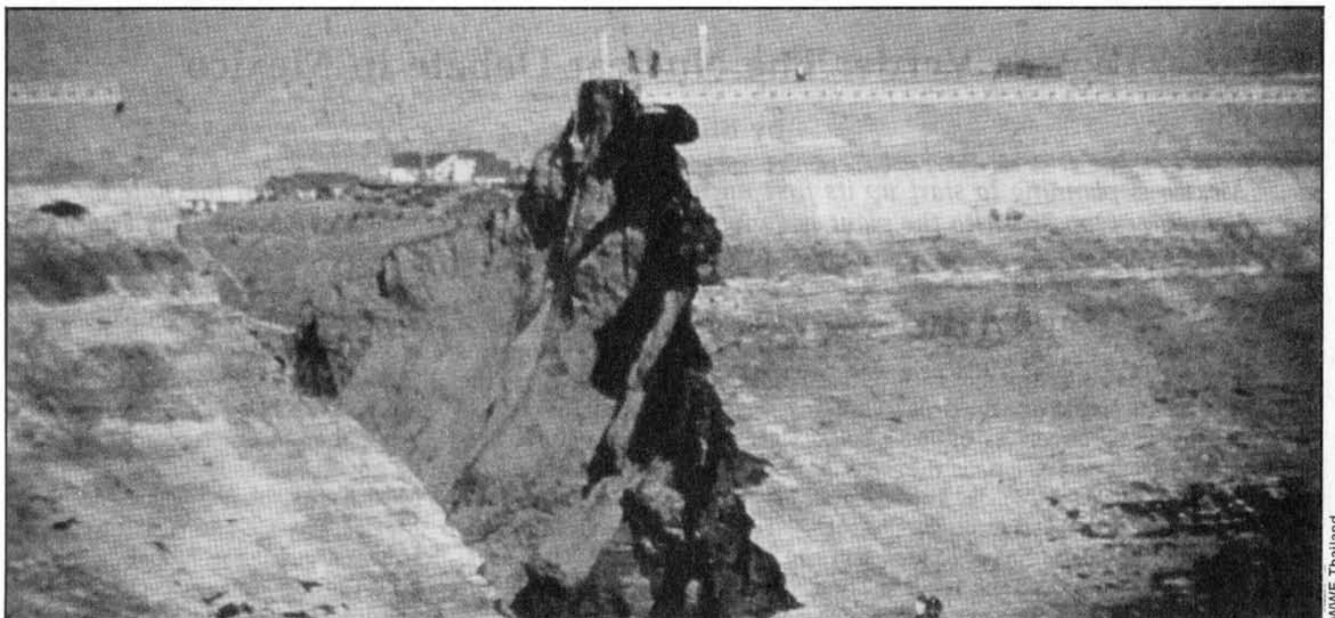
The Baldwin Hills Dam, damaged as a result of the movement of rocks along a fault line.
