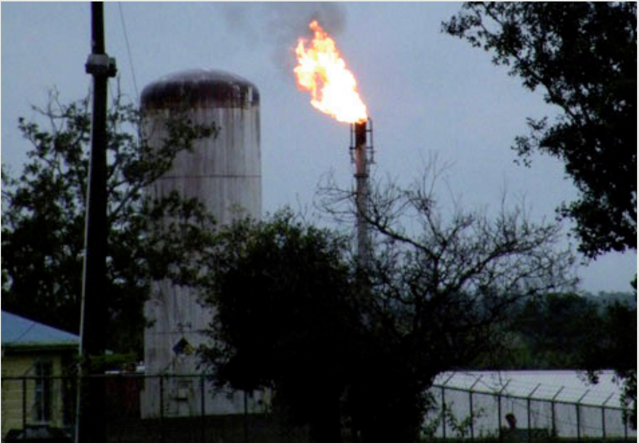
Flare at Spanish Lookout oilfield, operated by Belize Natural Energy with CHx investment. Photo: Robin Llewellyn
